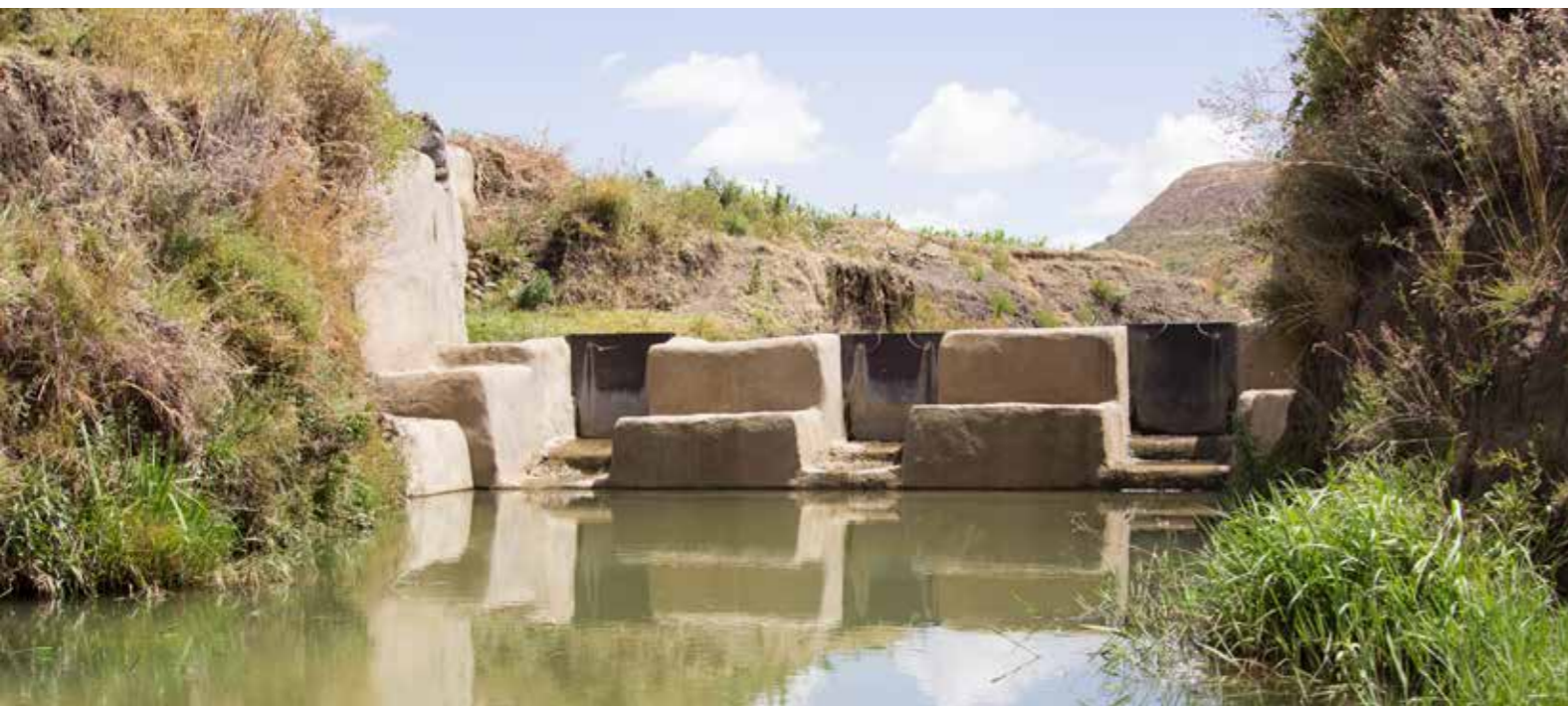
A check dam constructed in Tigray region in Norwegian Church Aid's climate resilience program. Together with various water harvesting schemes the project has proved to increase productivity in agriculture which has again improved livelihoods. The program is part of the national programme that has contributed to Tigray being greener than it has been in 145 years. The Tigray region has won several rewards, the latest being a U.N.-backed award for the world's best policy to combat desertification and improve fertility of drylands. Photo: Hilina Abebe, Norwegian Church Aid Ethiopia
